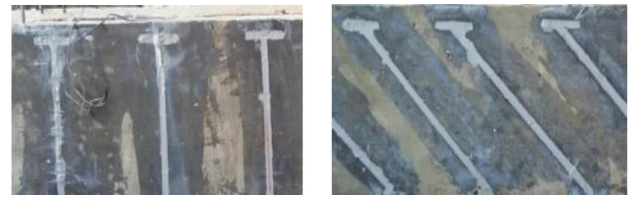
Fig. 3 the end anchorage
